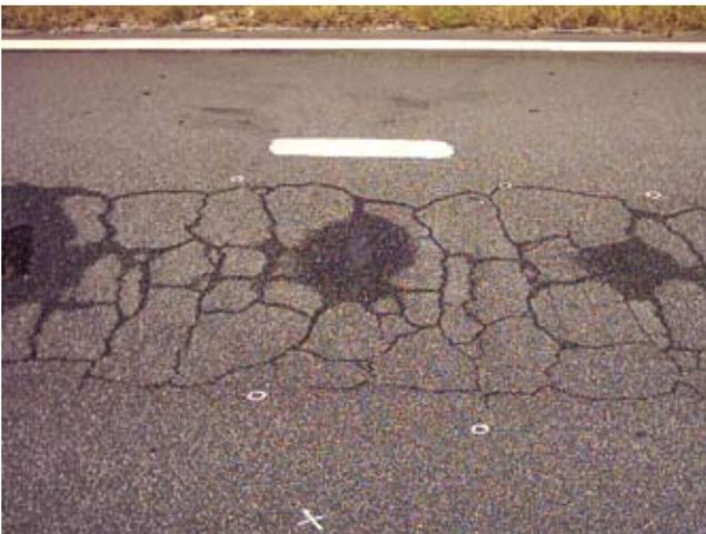
**Alligator or Fatigue Cracking** (Figure 5) — Interconnected cracks occurring in the wheelpath resulting from the applications of excessive traffic loads. These normally start as short transverse cracks occurring within the wheelpaths.
