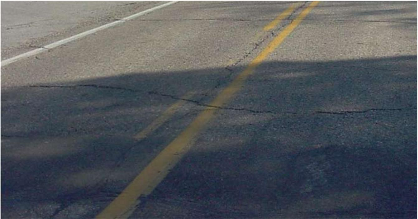
**Transverse Cracking** (Figure 4) — Cracking occurring at 90° to the direction of traffic, due to either the expansion and contraction of the pavement surface or as a result from cracks in lower layers reflecting through the surface.
