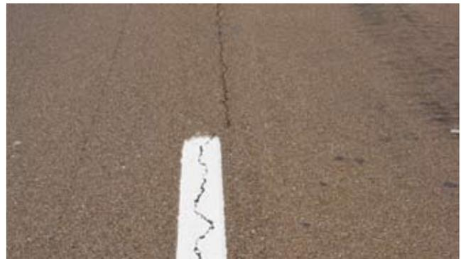
**Longitudinal Cracking in the Wheelpath** (Figure 3) — Cracking resulting from the application of traffic loads causing excess tensile strains. These cracks may originate either at the surface of the pavement or at the interface with the lower pavement layer.
